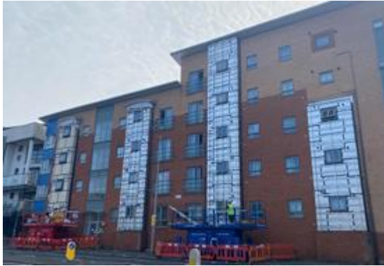
Progression on Elevation B
